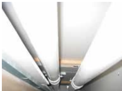
Photograph 1: Typical flue within a ceiling void
